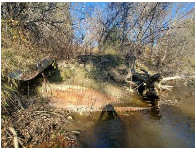
Figure 2-3: CSV Half-Pipe at the Edge of the Indian River (Looking Downstream)
