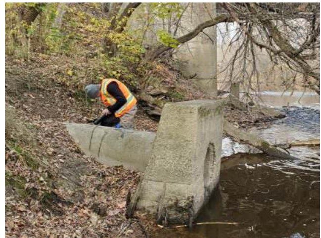
Figure 2-2: View of Outfall 41 Looking Downstream
