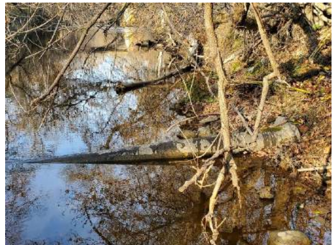
Figure 2-2: Cast Iron Pipe Extending into the Indian River (Looking Upstream)
