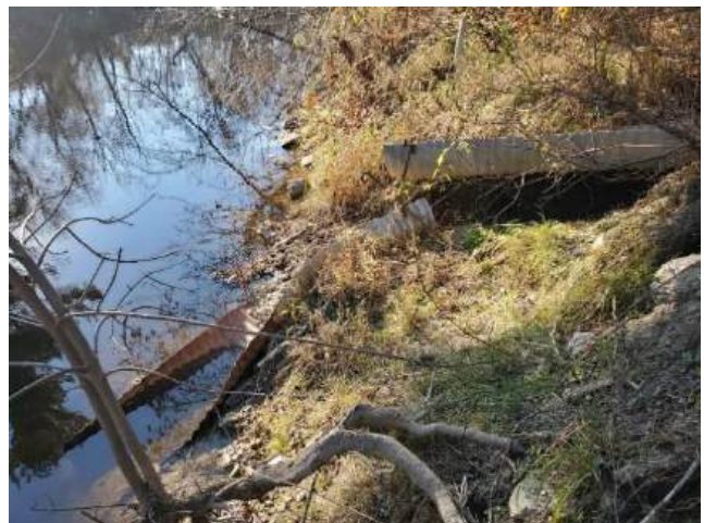
Figure 2-4: CSV Half-Pipe at the Edge of the Indian River (Looking Upstream)
