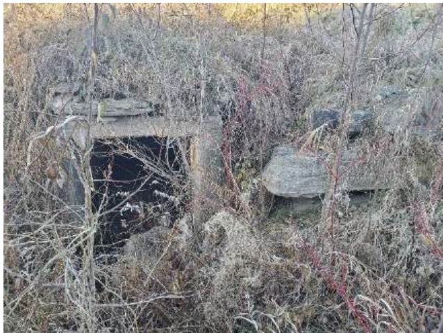
Figure 2-1: Box Culvert under the Asphalt Road (Box Culvert #1)
