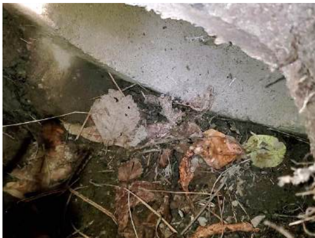
Figure 2-3: Close-up Photo of the Recessed Concrete Pipe Outlet
